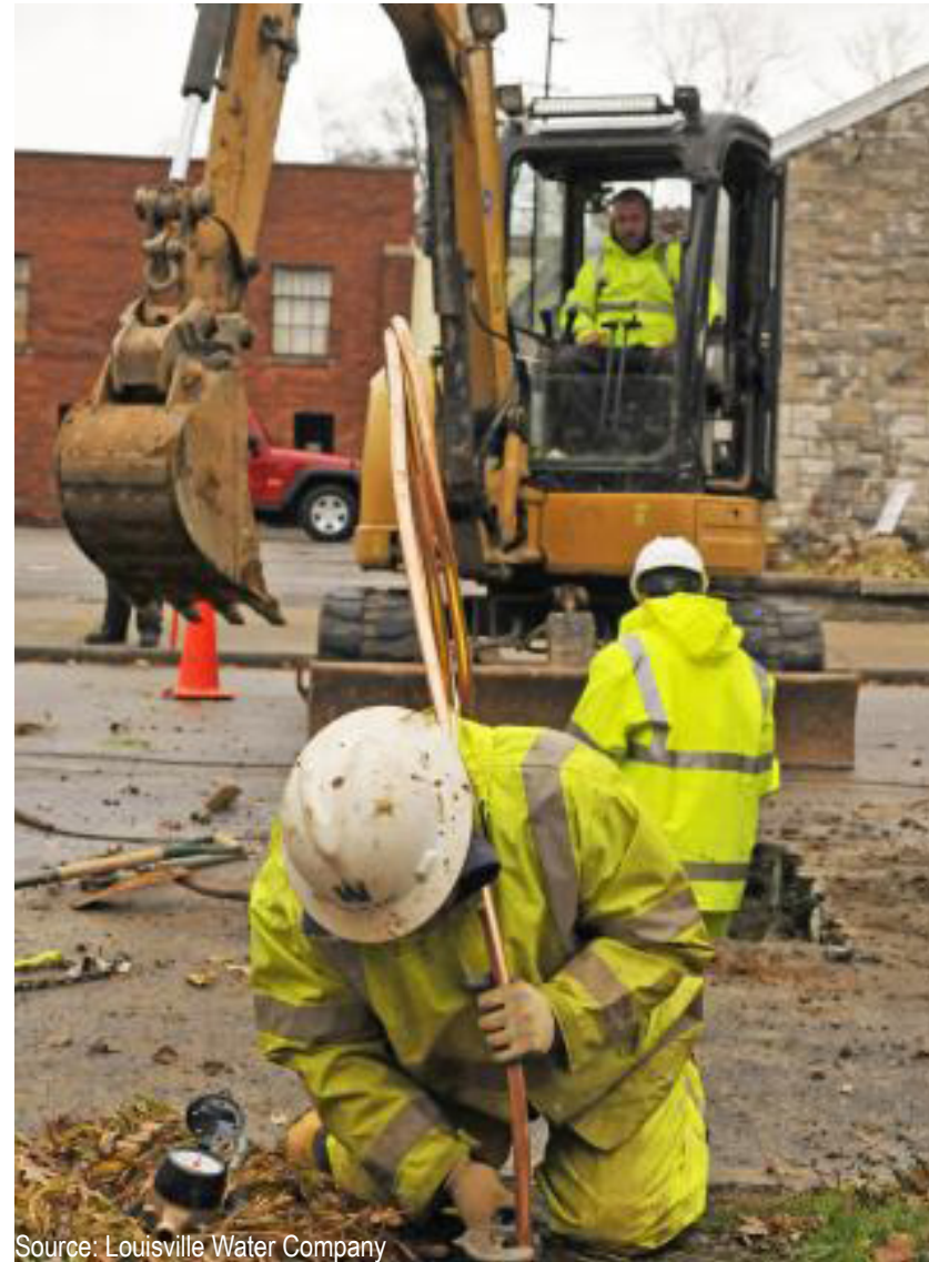
Figure 60 | Lead Line Replacement Program, Louisville Water Company
